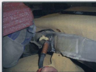
14. Weld ball joint mount
