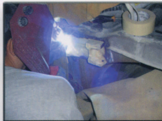
10. Remove door, weld complete
